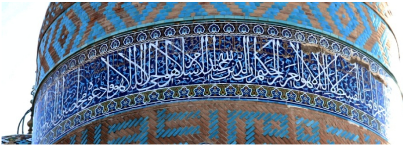
Figure 3 – Two Lined Band of Inscription Between the Body of the Tower and the Drum
